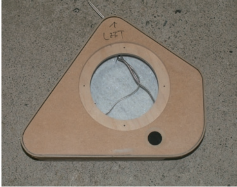
13. Place the surface panel onto the enclosure and make sure it fits
